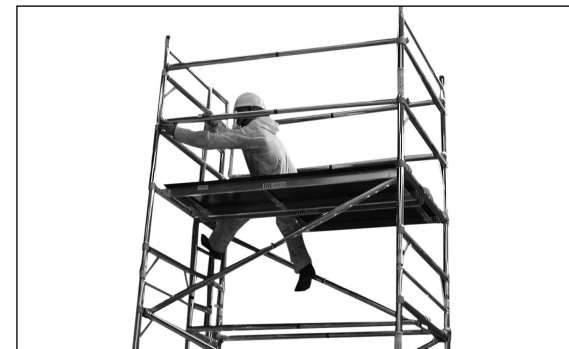
19 Dismantling is the reverse except when dismantling the handrails. Unclip the four end hooks and from the sitting position remove the handrails. Do not remove the handrails whilst standing on the platform, this would leave you at risk.
