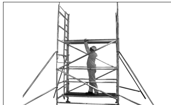
12 Fit trapdoor platform on appropriate rung above your head, see tower illustration guide.
