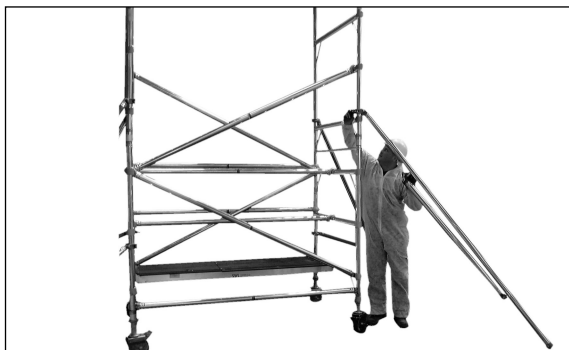
11 Secure stabilisers as soon as possible to increase tower stability. Check tower kit list to ensure the correct stabilisers are fitted.
