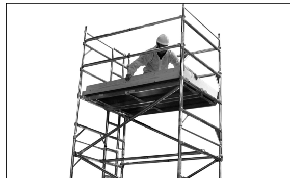
18 When handrails have been correctly fitted, fit toeboards.
