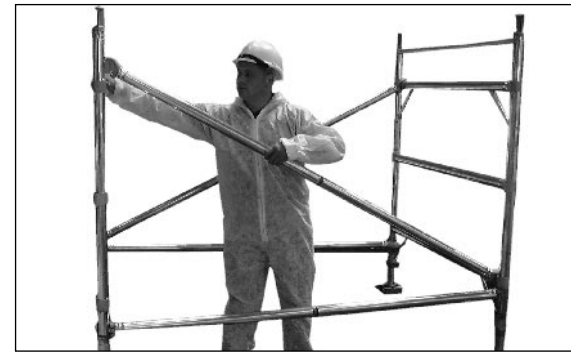
4 Klik in diagonal braces, starting at the bottom rung. Braces should be added in a continuous pattern. When fitting a full intermediate work platform it is permissible to interrupt the continuous pattern.
