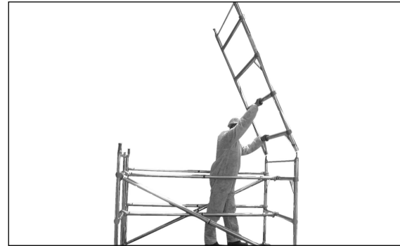
8 To add further frames, stand on platform ensuring the ladder frames are in line.
