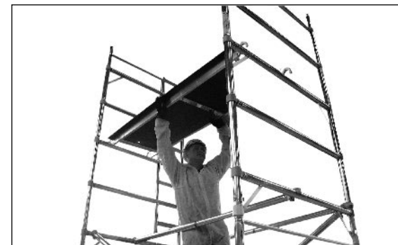
15 Remove plain platform from the bottom and reposition as shown.
