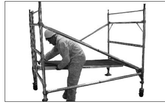
5 Fit plain platform on appropriate rung of frame. See tower kit guide for illustration. This will indicate which rung to fit trapdoor platform depending on final tower height.
