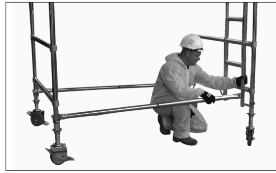
3 Klik in two horizontal braces to vertical member of the frame, as low down as possible.
