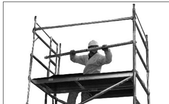
17 From the sitting position through the trapdoor (3T), fit four handrail braces to vertical member of frames.
