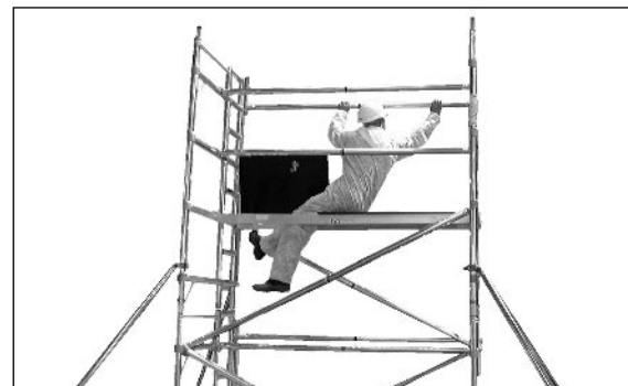
13 From the sitting position through the trapdoor (3T), fit four handrail braces, two on the outside and two on the inside as shown.
